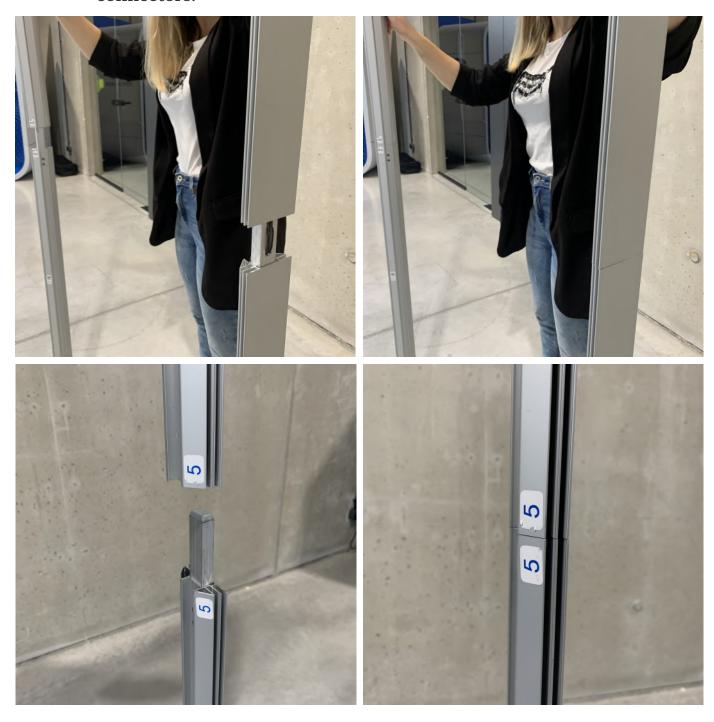
6. Install the LED courtain in the inner sleeve on the back of the frame. (Back is the side with two sleeves on the edges).
